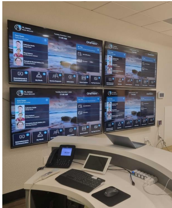
Oneview installation in Baxter's Customer Experience Center
